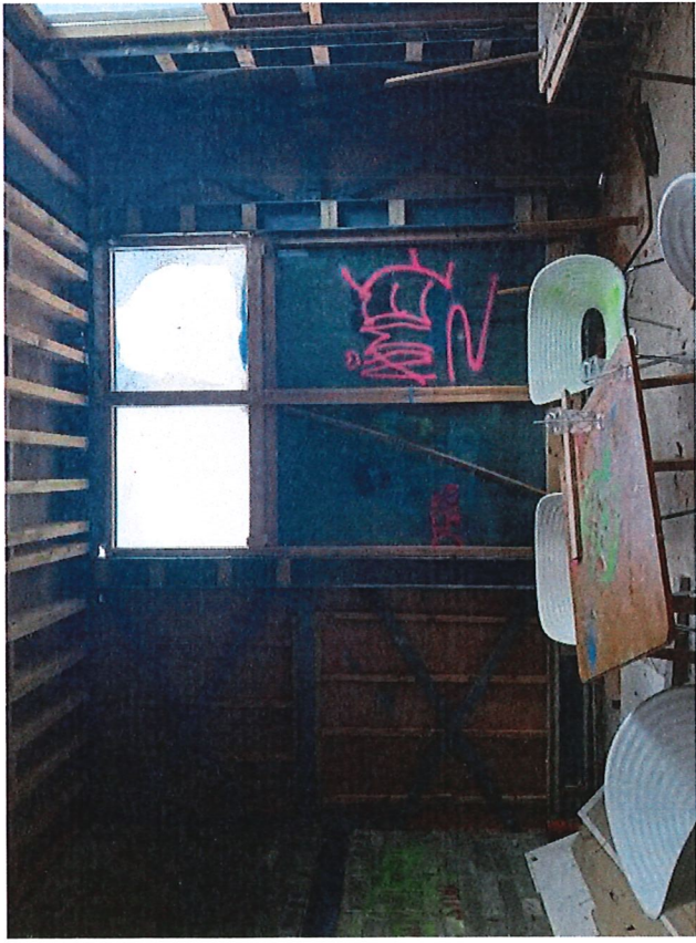
Fig. 49 – GF/06 – View south
