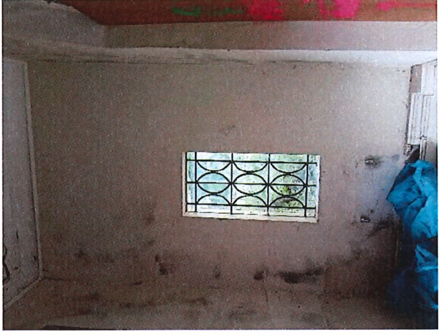
Fig. 32 – GF/01 – View west
