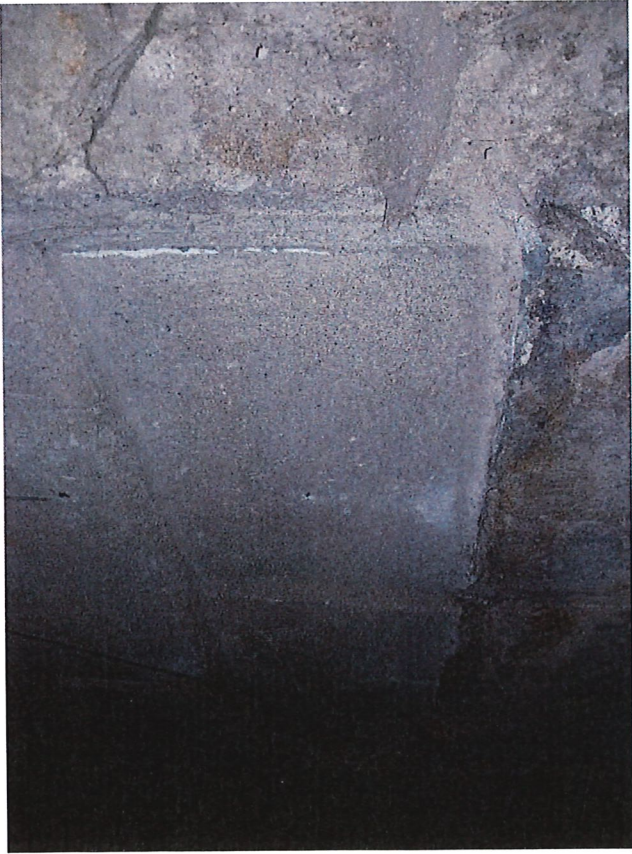
Fig. 9 – B1/02 – Detail ruled and lined cementitious render
