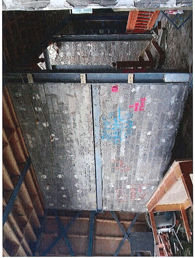
Fig. 48 – GF/05 – View east
